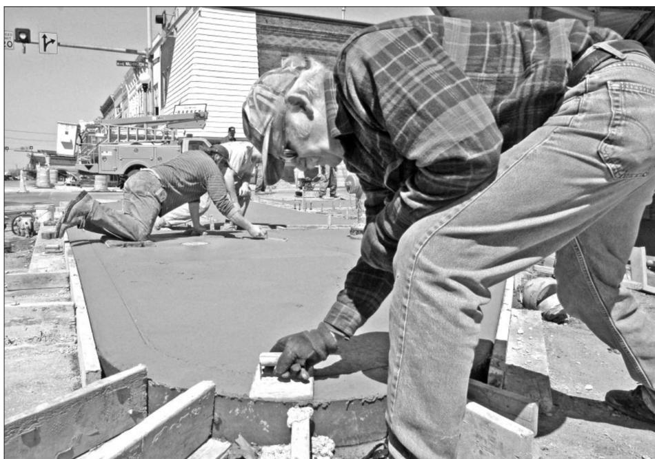
Workers lay cement as part of the sidewalk project on Franklin Street. The sidewalk project includes new lights, wider sidewalks and ramps compliant with the Americans with Disabilities Act.
